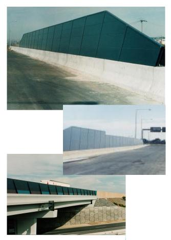
**GCS ACOUSTICS** designs and manufactures absorptive and reflective acoustic barriers for road and rail systems.
