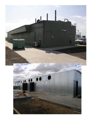
GCS Acoustics design, construct and erect Industrial plant rooms for many various applications. One of which is for prime power generators.
