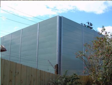
**GCS ACOUSTICS** design and manufacture absorptive and reflective acoustic walls for residential and industrial sites such as SEC Transformer stations.
