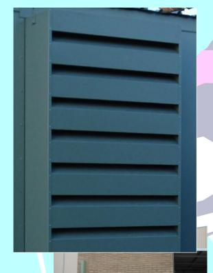
The GCS Acoustics Louvre has been designed to reduce noise levels when available area is restricted.
